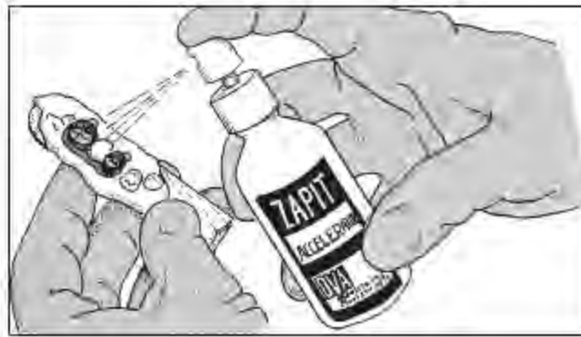
Fig 26-59 Zapit accelerator is sprayed into the joint.
